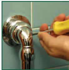
Install grab bars in the tub
